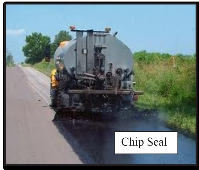
Figure 6: Chip Seal Treatment (21)
